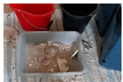
The top four photos show the roof, taken from above the ceiling. The bottom two photos show the main hall ceiling & fallen elements.
